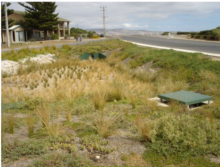
Figure 10.7 Bioretention Basin at Palmer Street, Aldinga Beach
