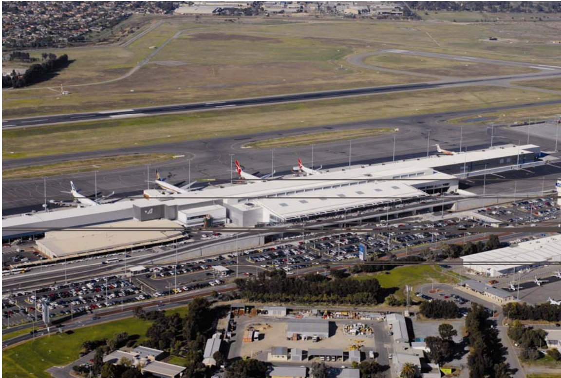
Figure 16.1 Adelaide Airport – One of South Australia’s Siphonically Drained Buildings
