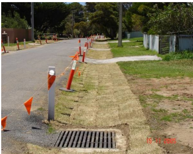
Figure 11.1 Palmer Street Swale Retrofit, Aldinga Beach
