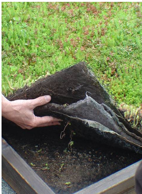
Figure 6.5 Extensive Roof Example
