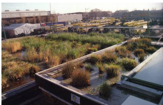
Figure 6.10 Constructed Wetland, John Deere Works, Germany
