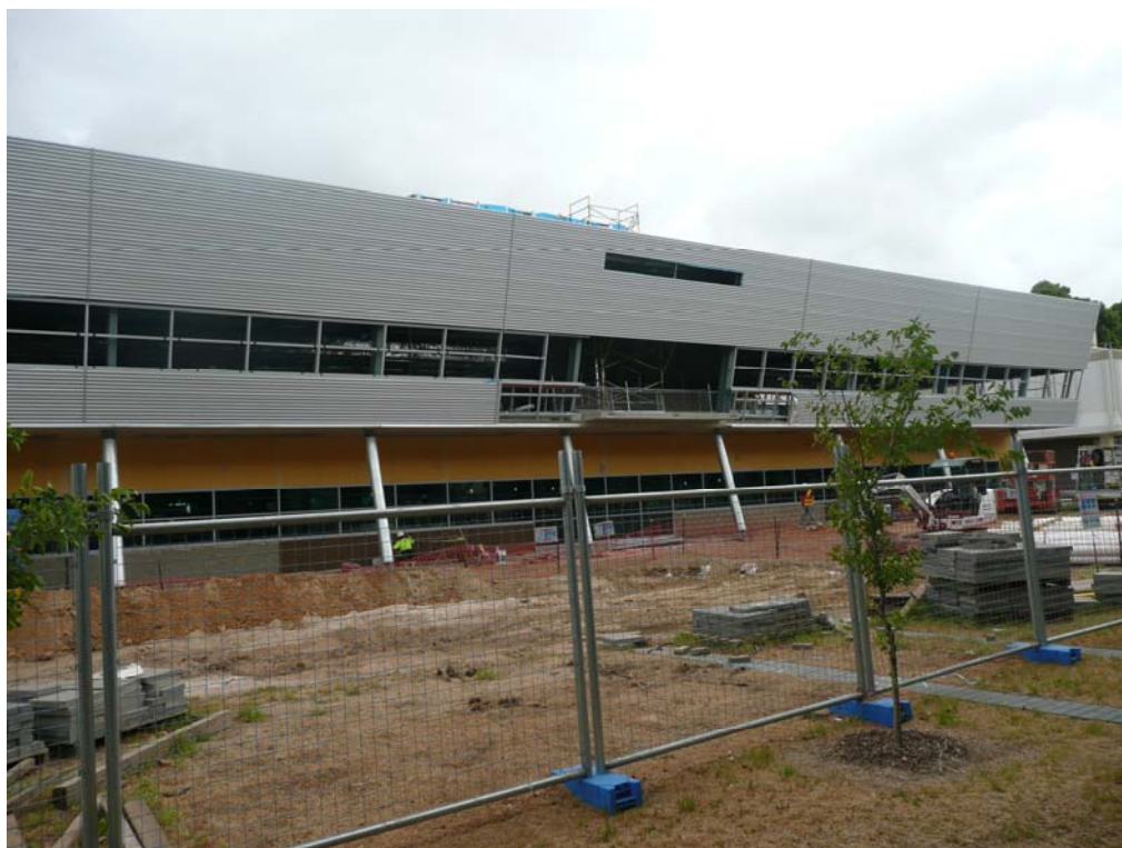
Figure 1.7 Construction of a New Building at Mawson Lakes Incorporating a Siphonic Roofwater Harvesting System
