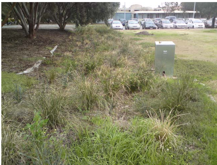
Figure 10.2 Bioretention Swale at Mawson Lakes Campus, University of South Australia (the swale also collects runoff filtered through a permeable paving system located in the carpark at the top of the picture)
