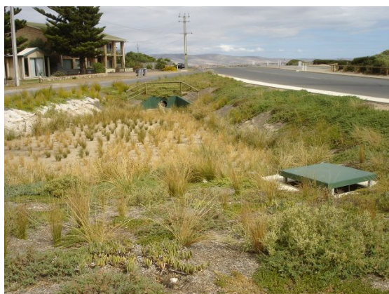
Figure 1.3 Bioretention Basin, Palmer Road, Aldinga Beach
