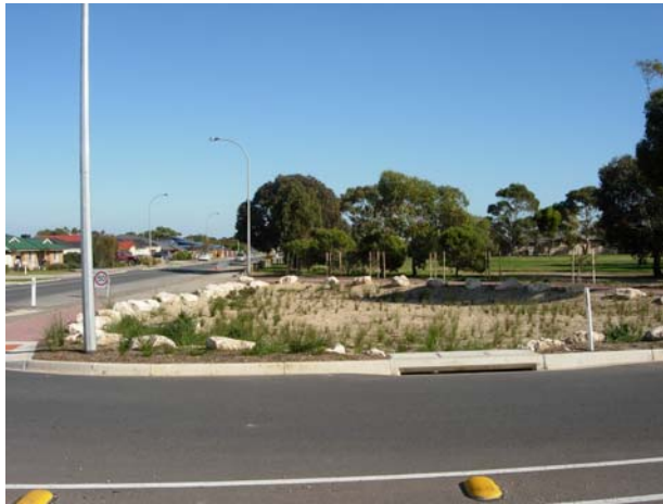
Figure 10.11 Alternative Pit Inlet Design for Depressed Bioretention Basin at Quinliven Road, Aldinga
