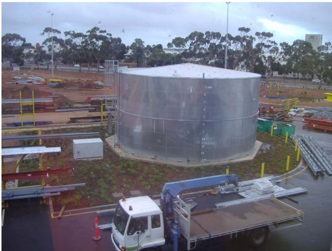
Figure 16.7 Rainwater Tank at the Bianco Warehouse at Gepps Cross
