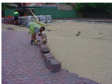
Figure 7.3 Construction of the Linden Gardens Car Park
