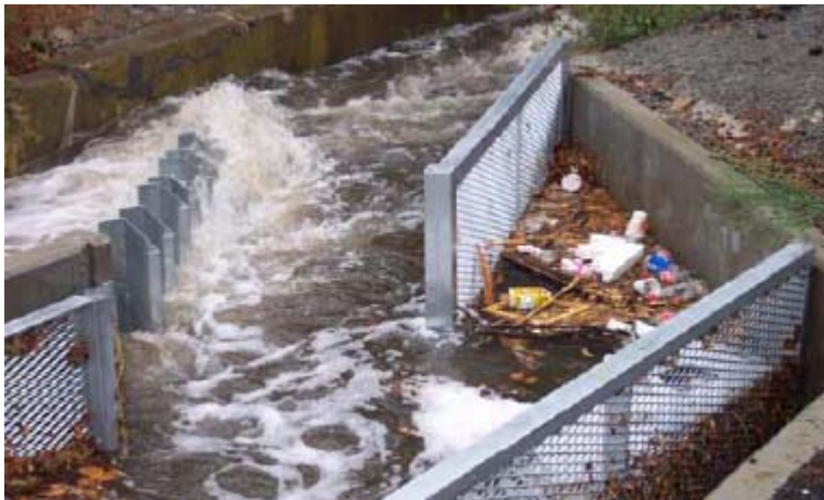
Figure 9.9 Vane Style Diversion Weir, Sebastopol, Victoria
