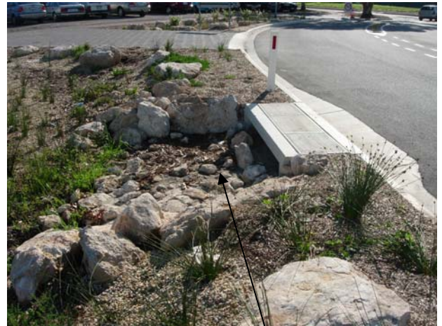
Figure 10.11 Alternative Pit Inlet Design for Depressed Bioretention Basin at Quinliven Road, Aldinga
