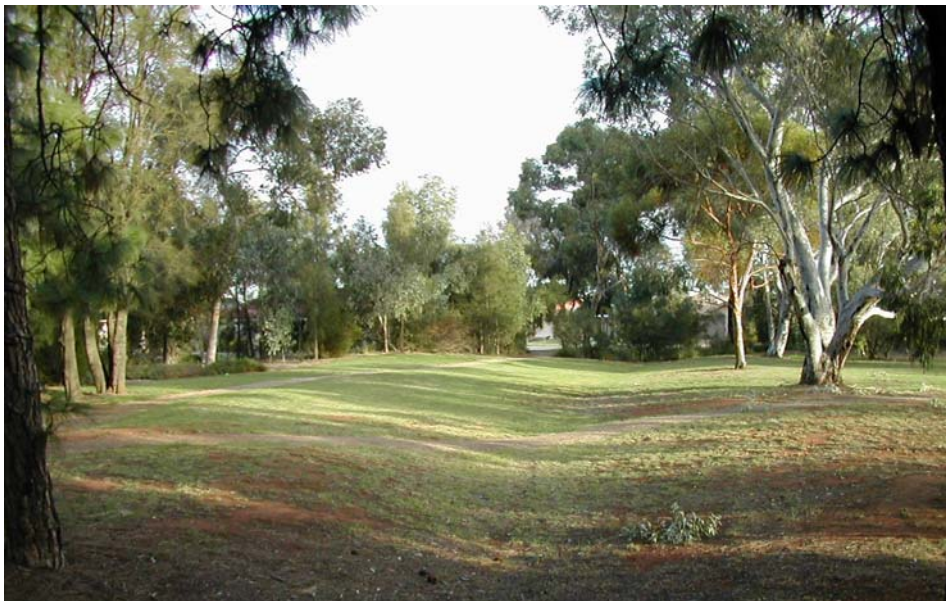
Figure 1.4 Swale at Pine Lakes, City of Salisbury
