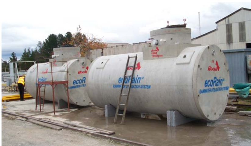
Figure 16.18: Installation of ecoRain Underground Rainwater Tanks
