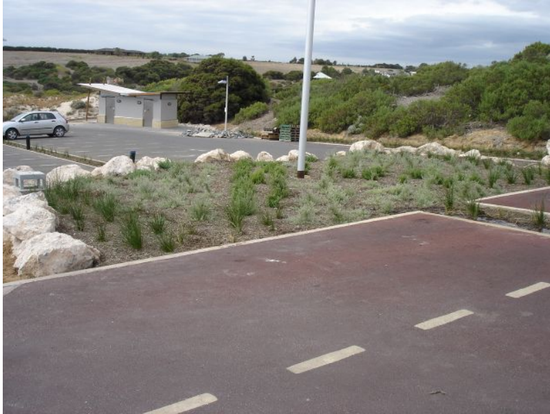
Figure 10.8 Bioretention Bed, Star of Greece Car Park
