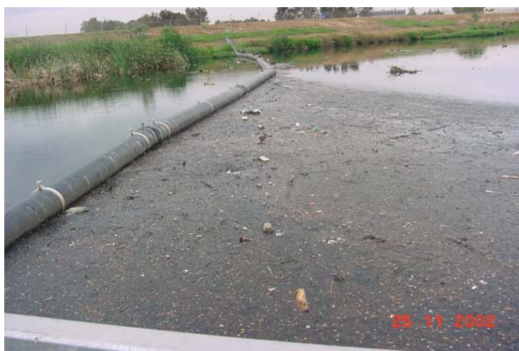
Figure 9.11 Floating Boom Operating at Netley, West Adelaide
