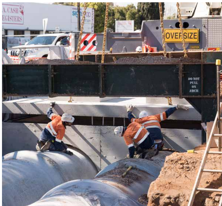
Trunk drain replacement and flood mitigation works in Port Road, Cheltenham
