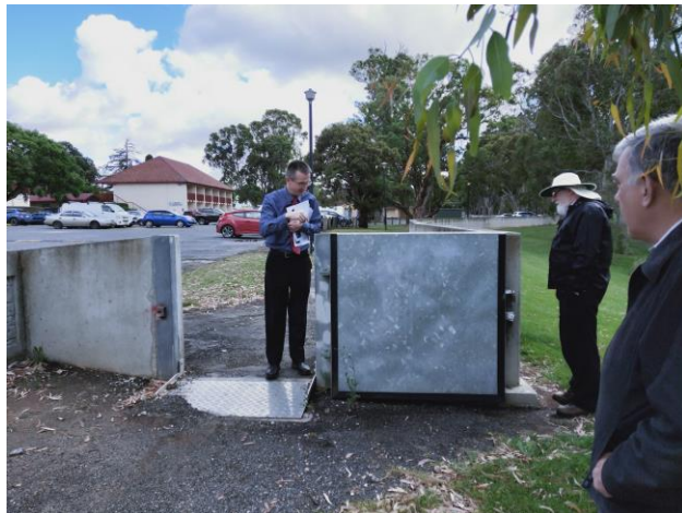
5 - A flood protection barrier gate which is closed during higher river flows.
