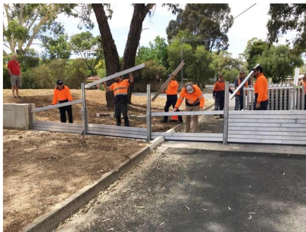
3 - The demountable barriers are easy to put in place.
