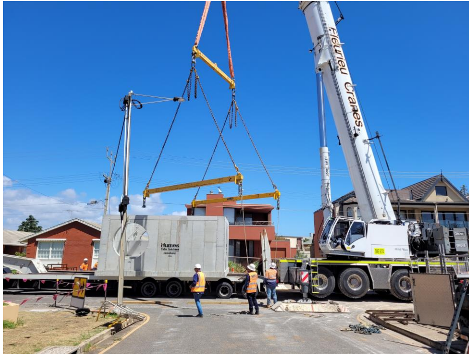
1 - Installation of a similar gross pollutant trap at Wattle Street, Hove.
