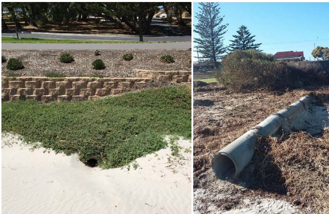
Figure 5.5—Drainage Outfalls at Semaphore South, Before and After Wave Action
