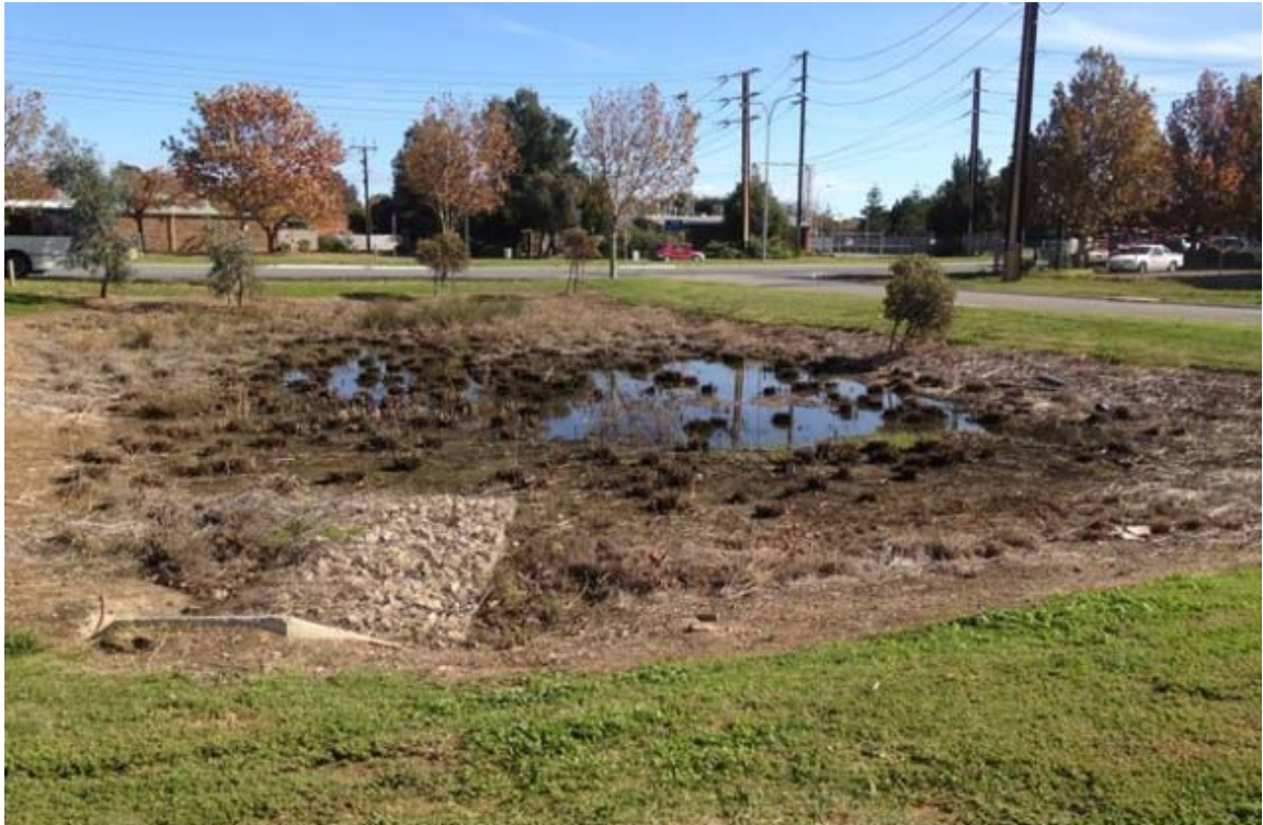
Figure 5.6—High Groundwater Level in the Mascotte Street Retention Basin
